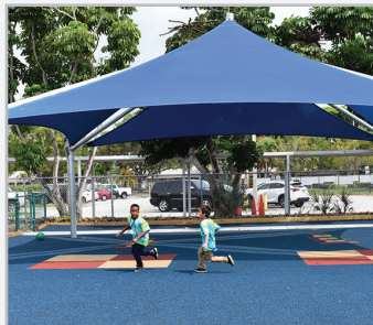
MAPLEWOOD ELEMENTARY SHADE STRUCTURE
